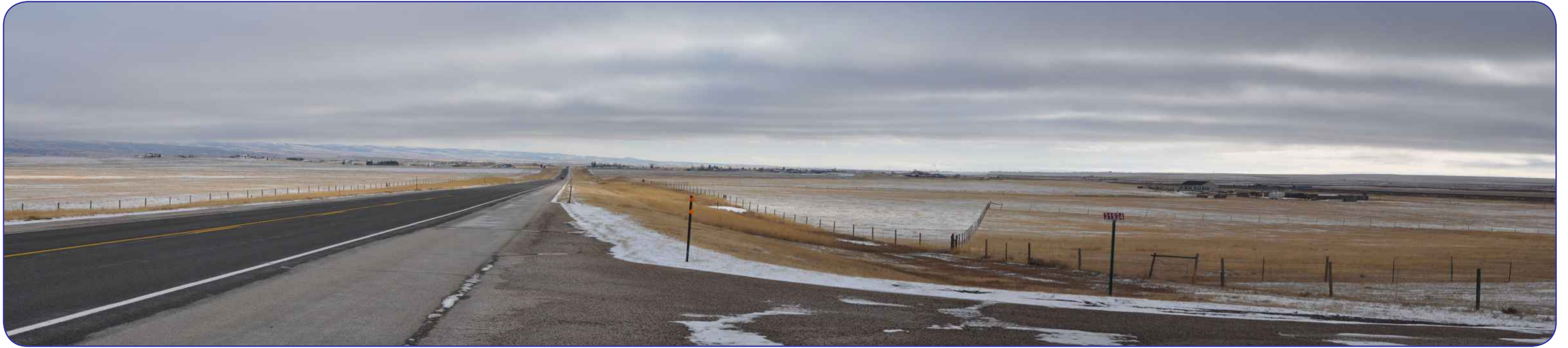
21. US 30 / South of Oasis Ranch Road - Views looking south-southwest
