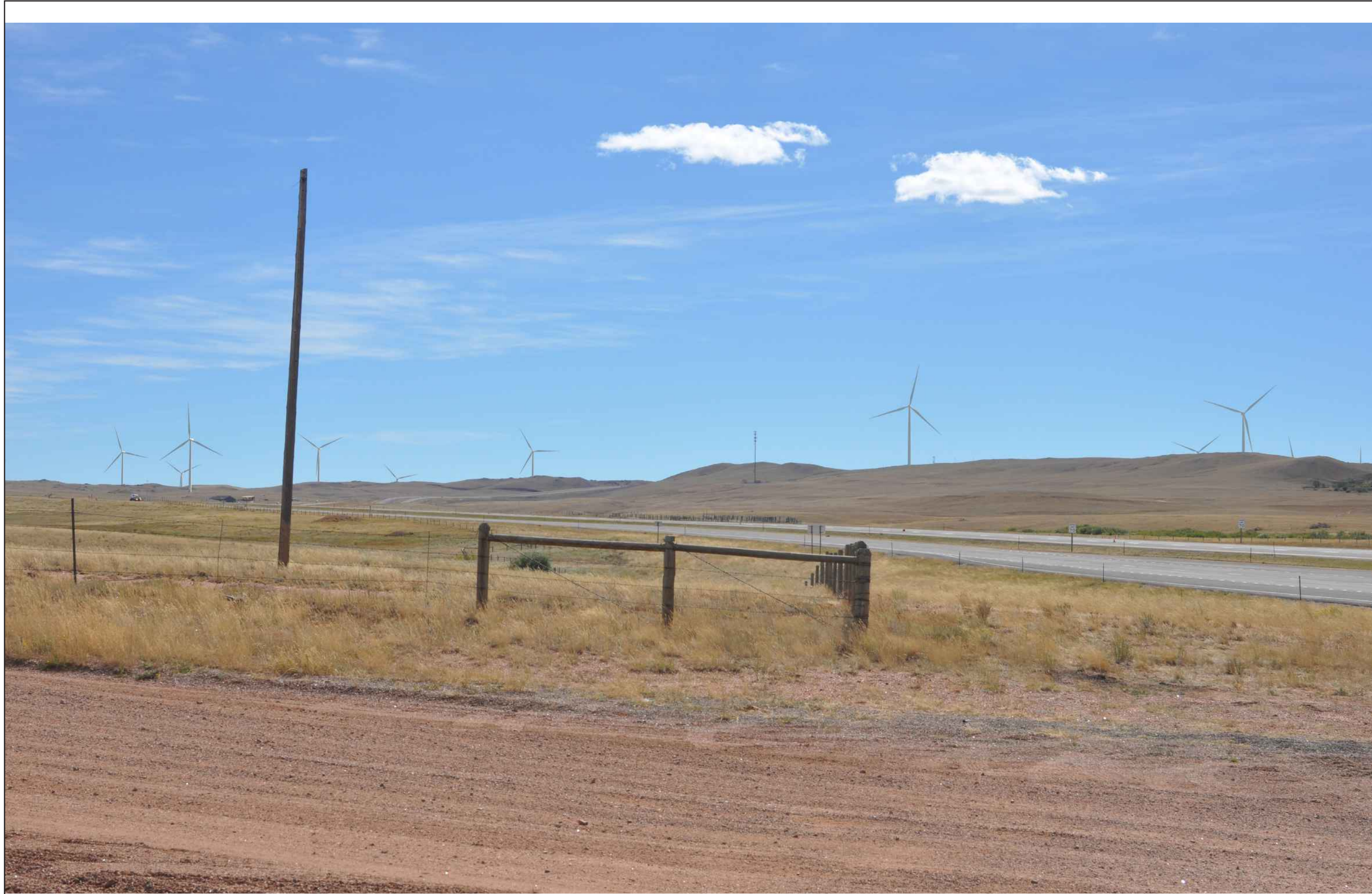
KOP001 Tie Siding Early Afternoon, viewing Southeast GE 3.0MW, Minimum Turbine Height Scenario
