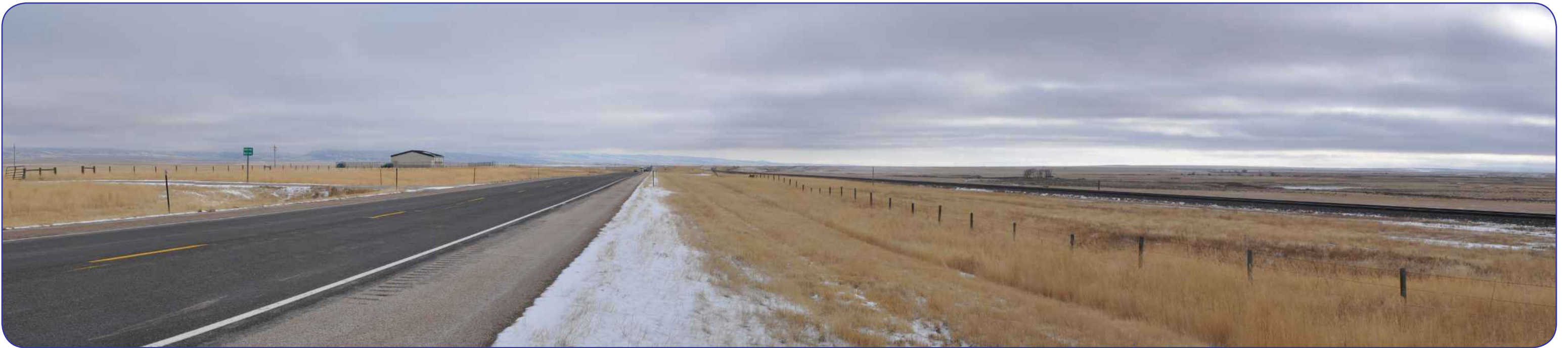
22. US 30 / Zog Road - Views looking south-southwest
