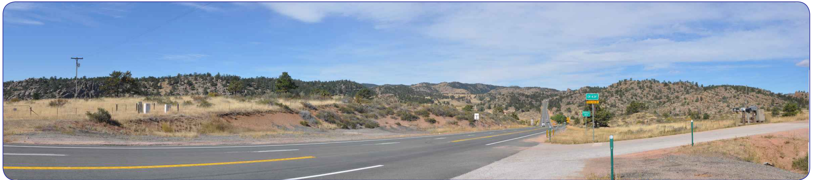
10. Virginia Dale Monument - Views looking northwest
